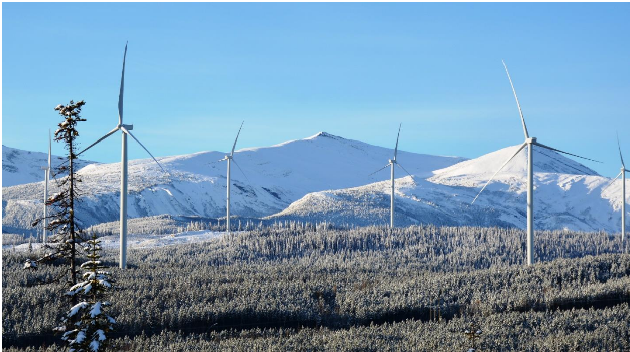
Pattern Development's Meikle Wind Power Facility
